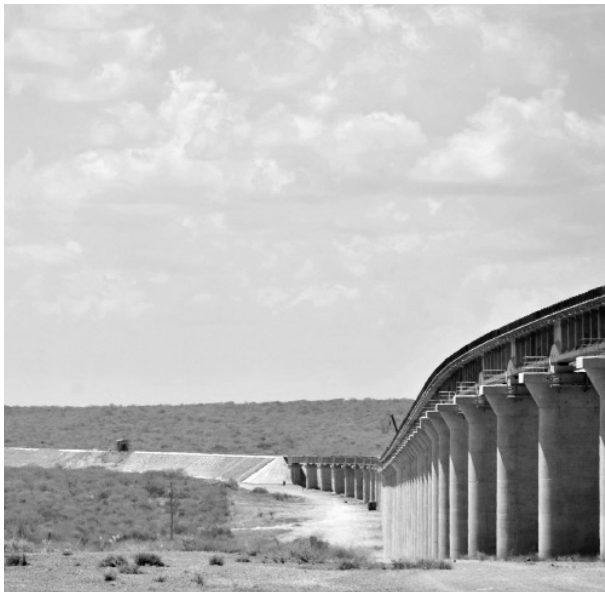
Figure 9: Part of the section of the Standard Gauge Railway cutting through Tsavo National Park.
